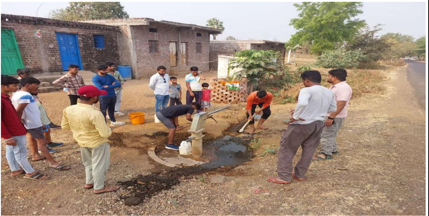
NSS volunteers constructing drains around the hand pump of the village under the special camp of NSS.
